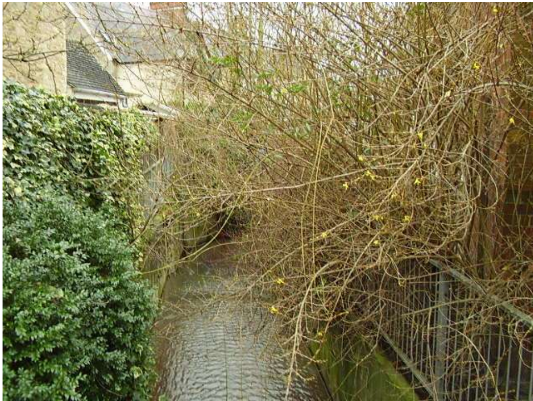
Area 5 – Madley Brook View looking downstream of culvert C09
