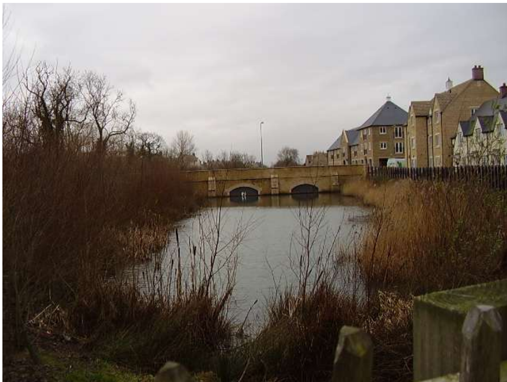
Area 5 – Madley Brook View of upstream balancing lake near Harvest Way and Culvert C04
