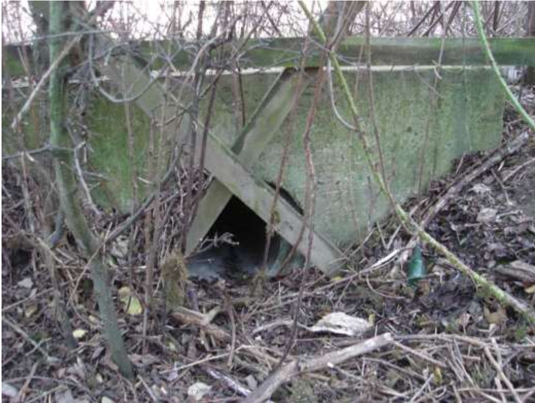
Area I3 View of Culvert 14 under A40
