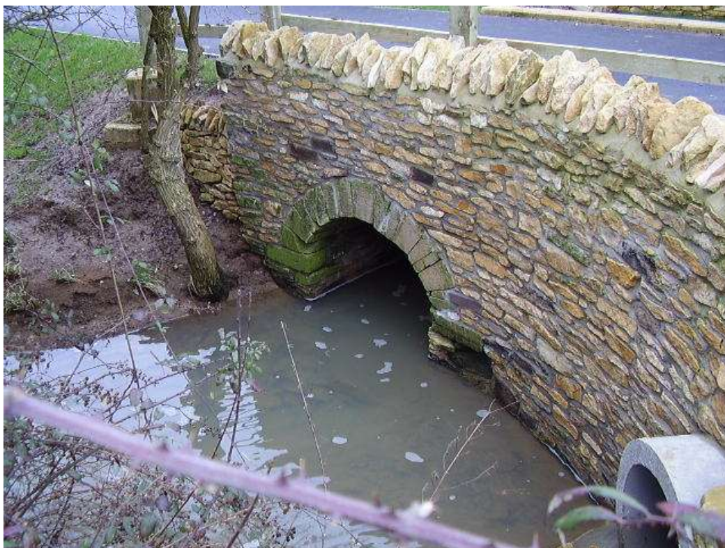
Area 5 – Madley Brook Downstream view of culvert C05
