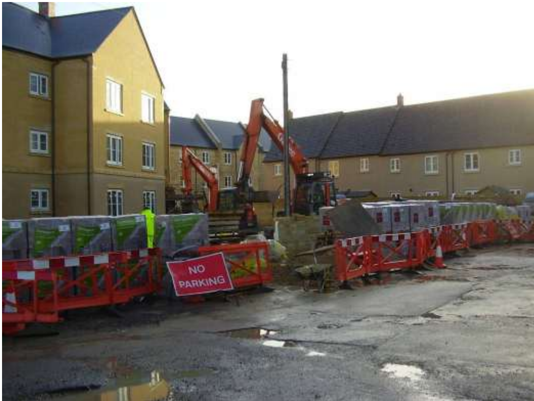
Area 6b Construction of Aquarius behind the houses along Bridge Street.(05-12-08)
