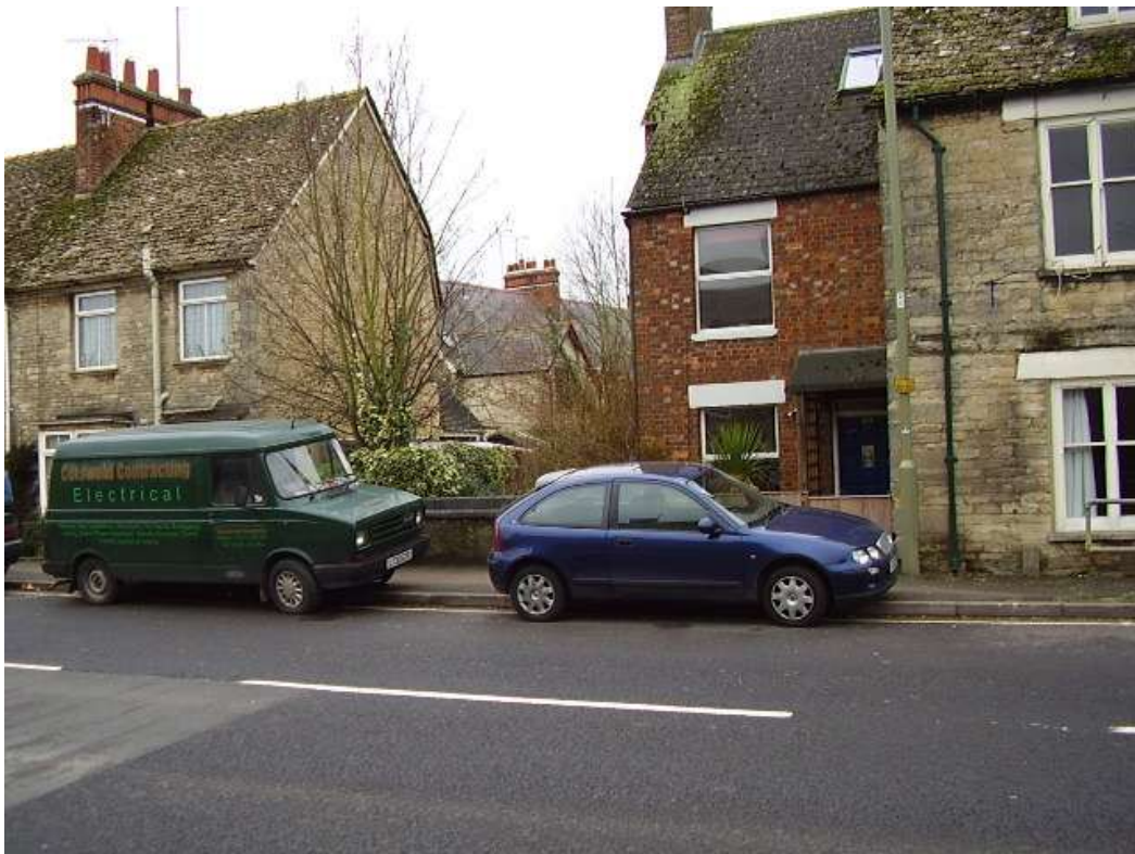
Area 5 – Madley Brook View looking across culvert C09 from upstream to downstream
