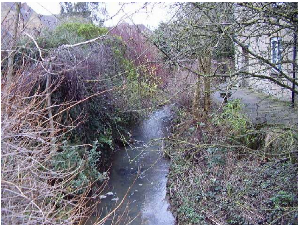
Area 5 – Madley Brook View looking upstream from culvert C09
