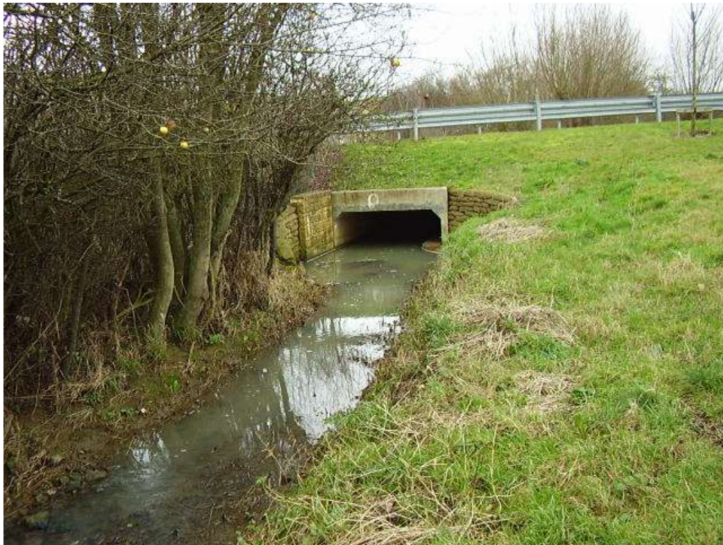
Area 5 – Madley Brook Downstream view of culvert C04 under Madley Way
