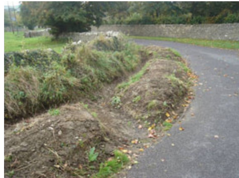
Area I – newly cleared grips and ditches to south - east of Swin Lane
