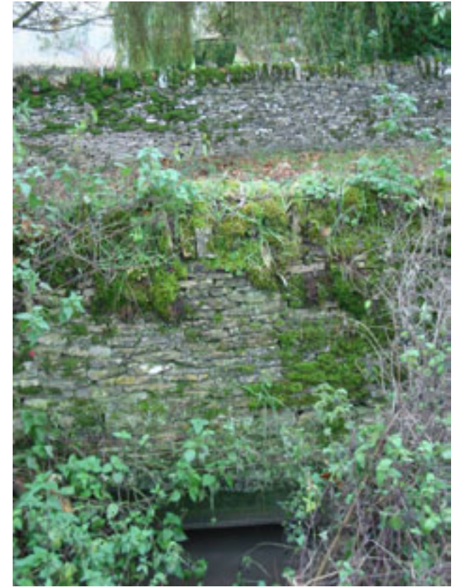
Area 3 – culvert carrying watercourse under the highway
