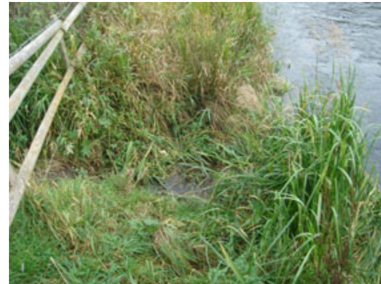
Area I – junction of watercourse with River Windrush
