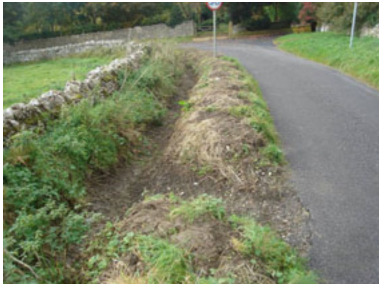
Area I – newly cleared grips and ditches to south - east of Swin Lane
