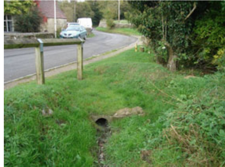
Area I – culvert outlet to ditch opposite the Swan Inn
