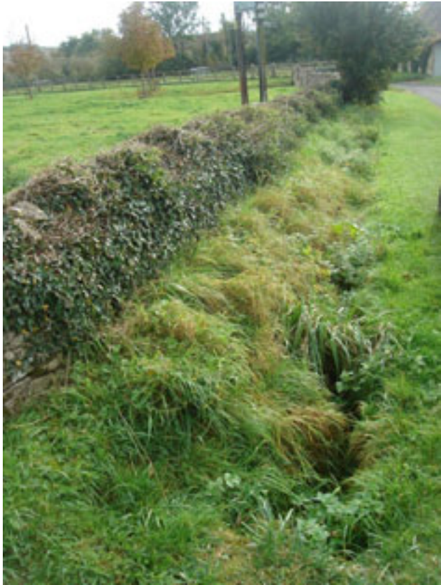
Area 1 – Blocked ditches along route of watercourse, in contrast to newly cleared grips and ditches
