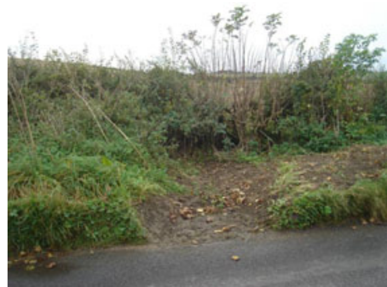
Area 2 – Asthall road, showing verge grips falling towards road
