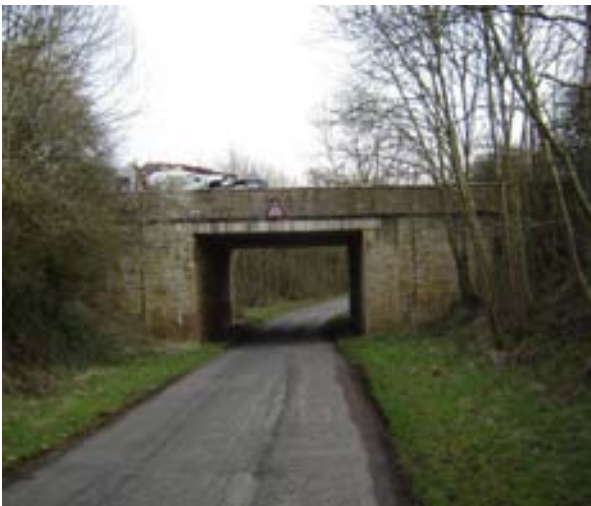
Area 5 - A361 over bridge over Little Barrington Road
