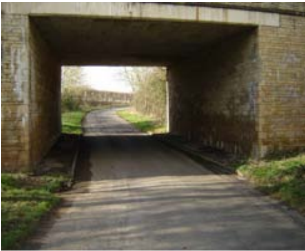
Area5 - A361 over bridge at Little Barrington Road
