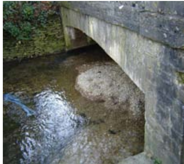
Area 3 - Thoroughfare bridge over Broadwell Brook
