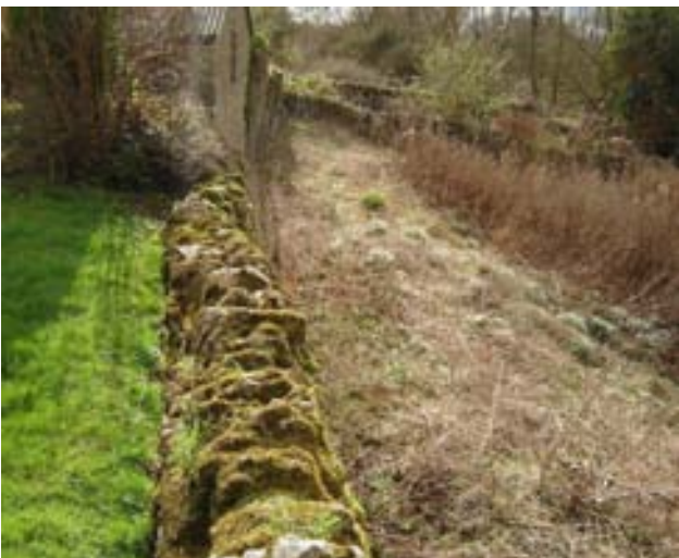
Area 2 – Attenuation location next to Meadow Cottage
