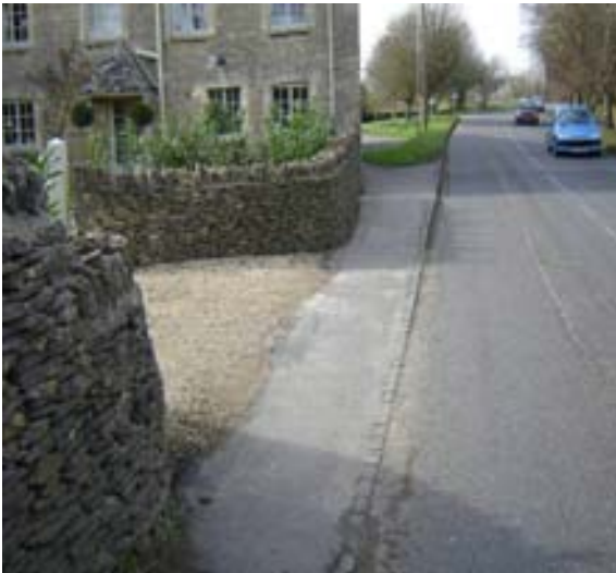
Area 8 - Low kerb face at Broughton Poggs
