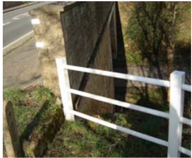
Area 5 - A361 Bridge over Barrington Road
