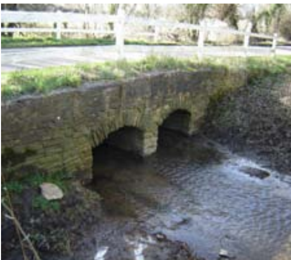
Area 6 - Broadwell Brook bridge at 'Goodfellows'
