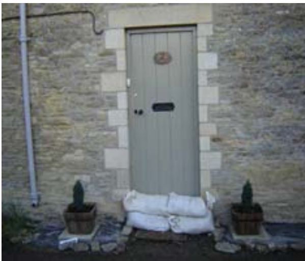
Area 3 - Threshold flood protection at Filkins
