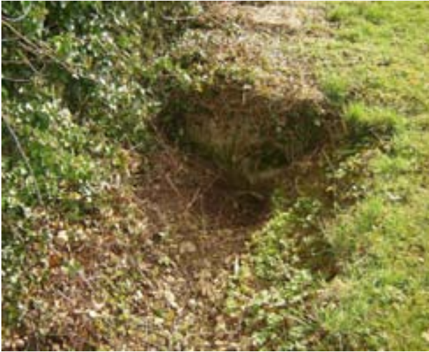
Area I - Culvert at Clark's Barn
