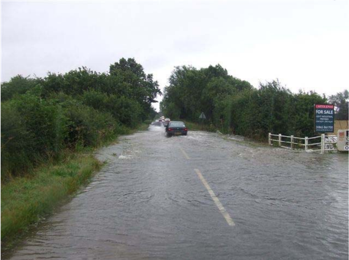
Station Road (Brize Norton to Bampton Road) – flood water flowing over road
