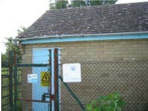
Area I - Thames water pumping station The Green
