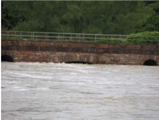
Area I - Railway bridge flooding
