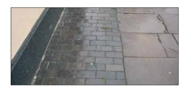
Traditional vehicle crossover surfaced with an irregular grid of stone setts; and a modern interpretation using concrete block paviours.
