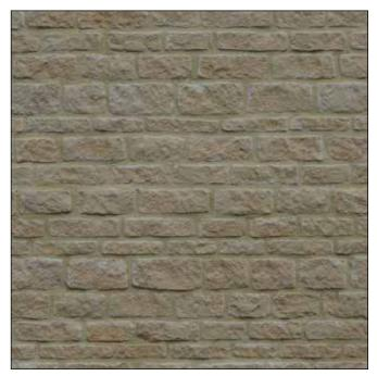
Fig. 8 Artificial stone wall
