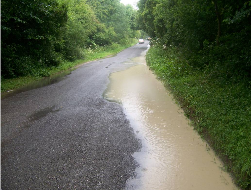
Photo 2 - The same section of road, looking towards East End. Where the road dips, the runoff collects in a ditch in the eastern verge,
