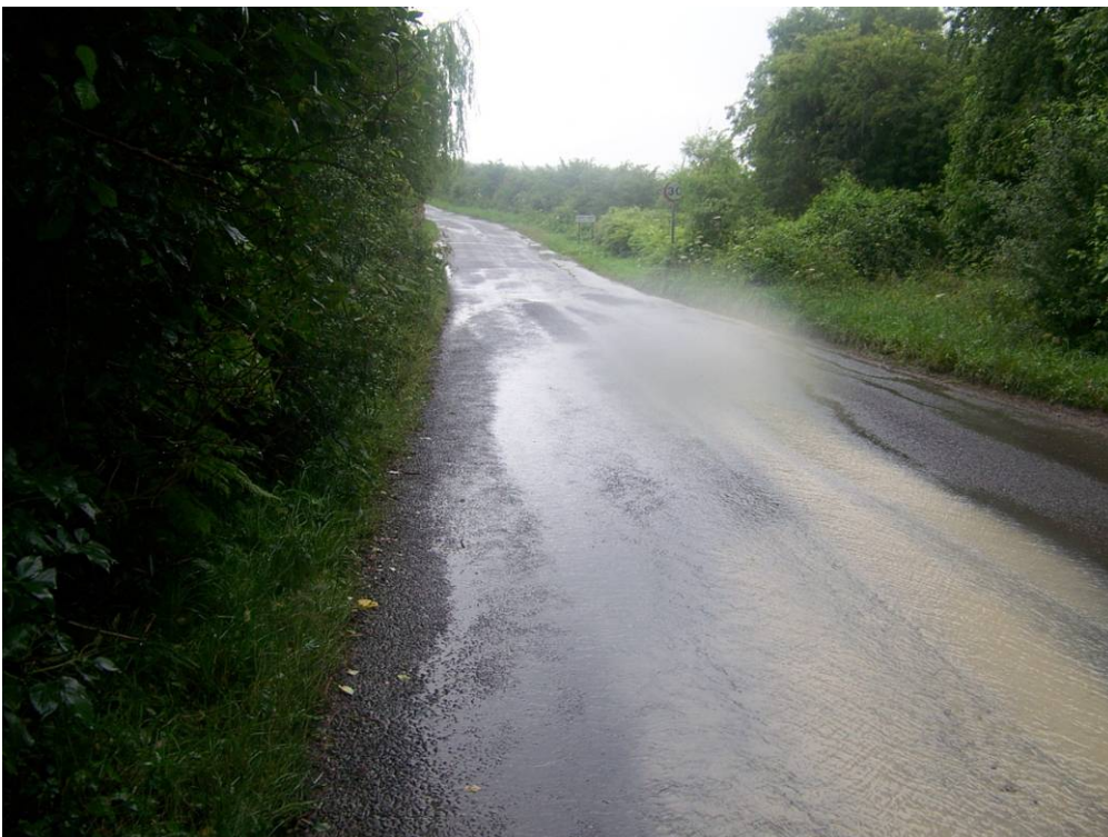
Photo 2 - The same section of road, looking towards East End. Where the road dips, the runoff collects in a ditch in the eastern verge,
