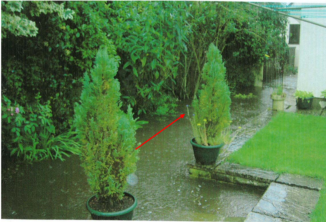
Photo 7 - As the above ditch surcharges, water follows the natural flow path through property on East End lane
