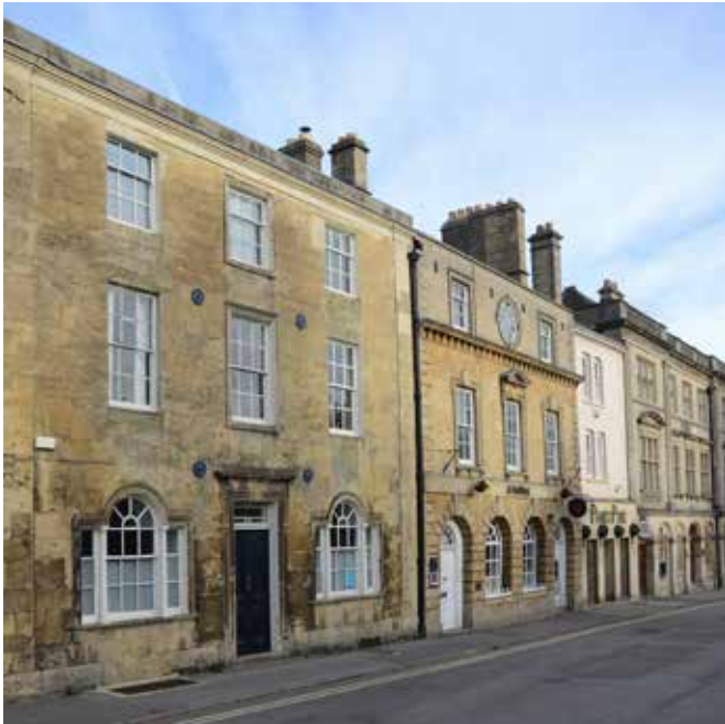
Formal built character on western side of Market Place
