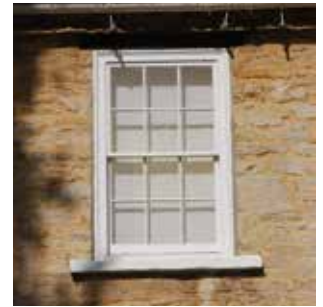
Traditional local timber sash and casement windows
