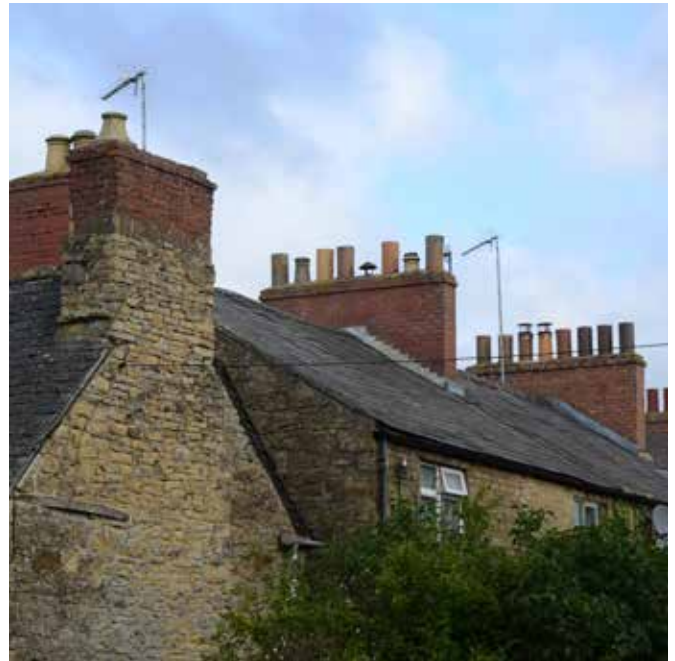
Brick and stone chimneys, and Welsh slate
