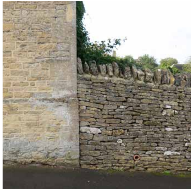
Local stone walling - both dressed and mortared, and dry
