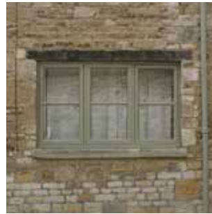
Traditional local timber sash and casement windows
