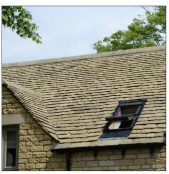
Fig. 7 Artificial stone slate roof with flush roof-light
