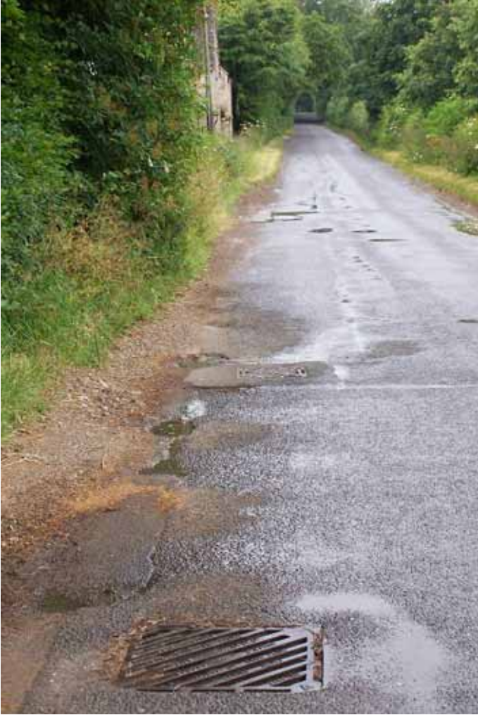
Photograph 25: Drainage along road, looking away from Shilton
