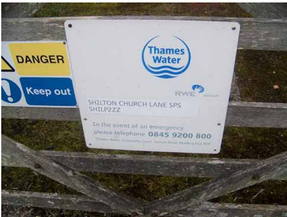
Photograph 20: TW sewage pumping station
