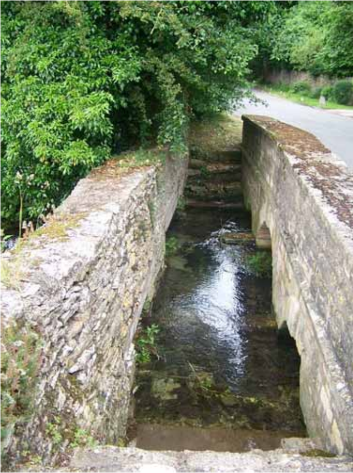
Photograph 7: Bridge Street Bridge upstream face
