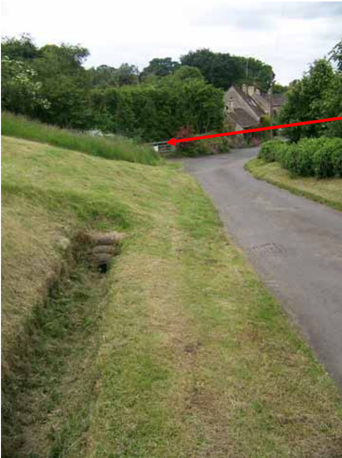
Photograph 19: Drainage ditch downstream end of Shilton, looking towards TW pumping station
