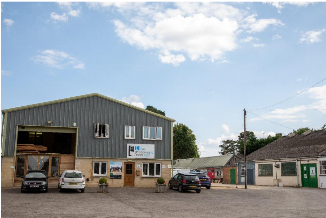
Groves Business Park in the centre of MuW with units of differing sizes
