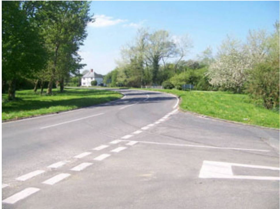
Photo 3 - Junction with Station Road – village green on right, looking towards Alvescot
