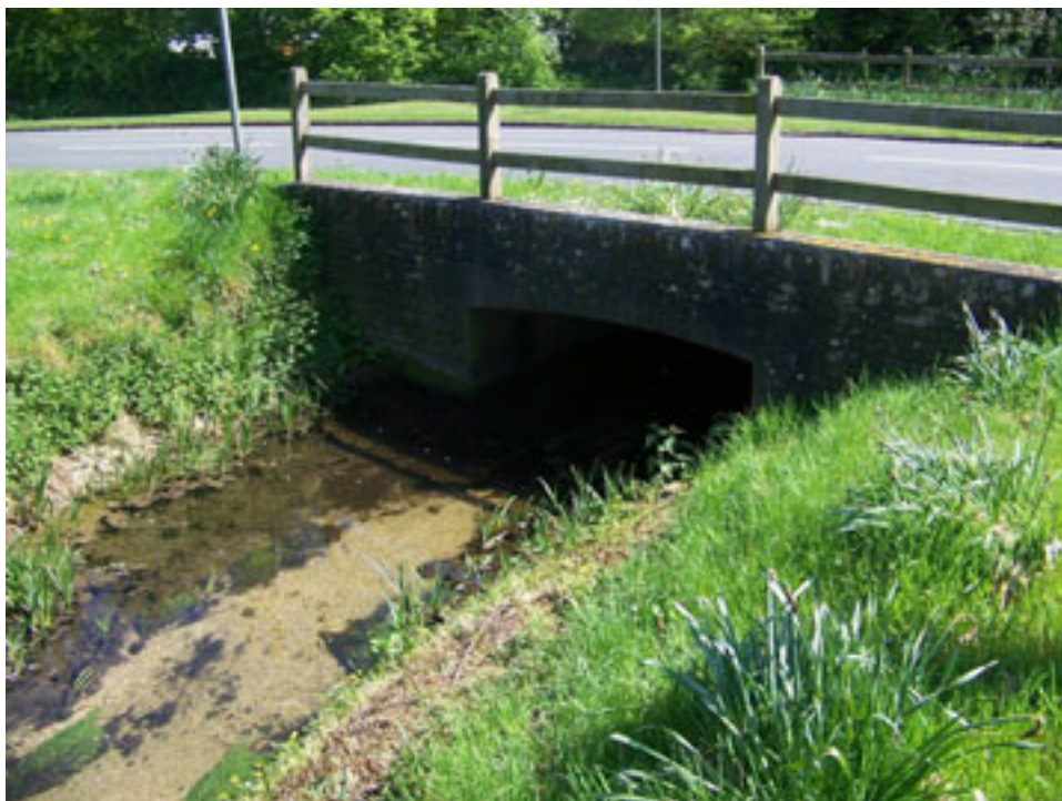
Photo 2 – Station Road Bridge at village green
