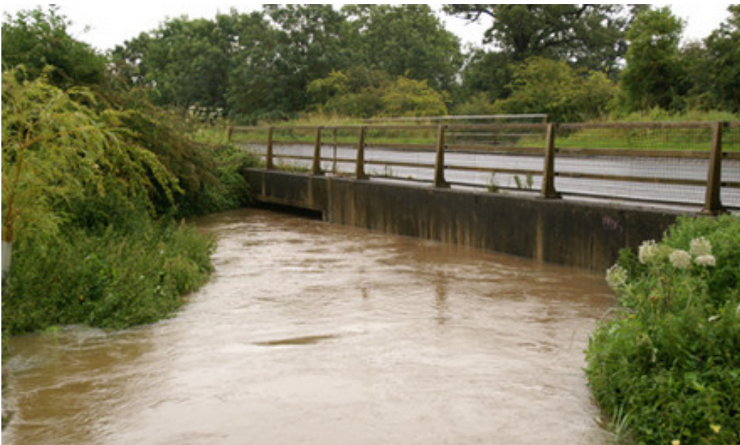
Photo 22 – B4449 bridge crossing July 2007
