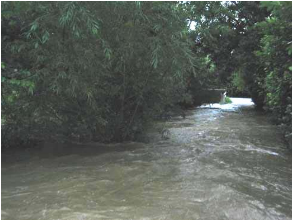
Photo 11 – Old A40 road bridge June 2007 – water is over the lane and bridge is surcharged.
