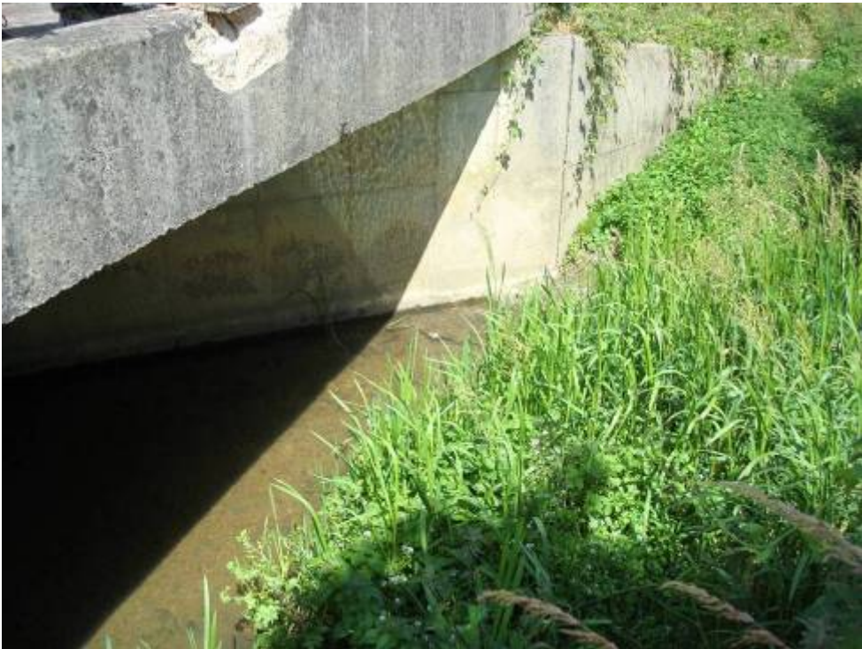
Photo 25 – Downstream face of B4449 road bridge
