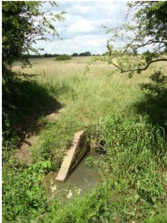
Photo 14 – Upstream face of Chil Bridge
