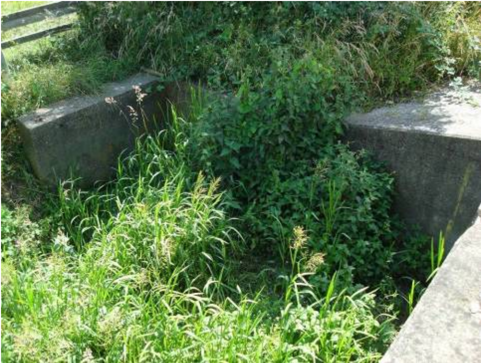
Photo 26 – Downstream of B4449 road bridge.
