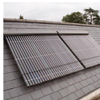
Fig. 28 Solar thermal panels - evacuated tube type
