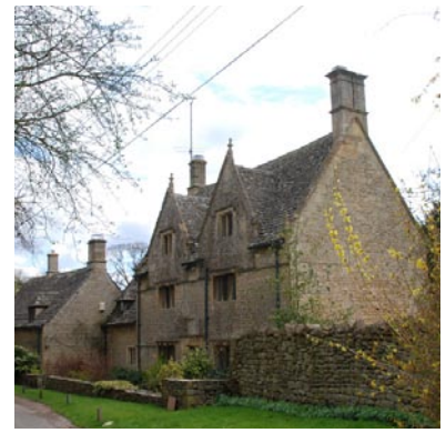
Fig. 13 Steeply-pitched traditional roof
