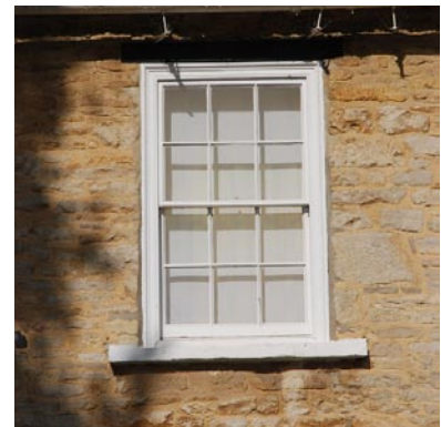
Fig. 10 Vertical sash window
