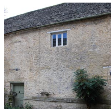
Fig. 12 Small window area in traditional house
