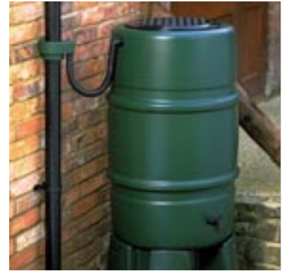
Fig. 27 Water butt for rainwater harvesting
