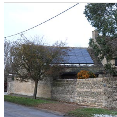
Fig. 29 Visually prominent photovoltaic panels on traditional building
