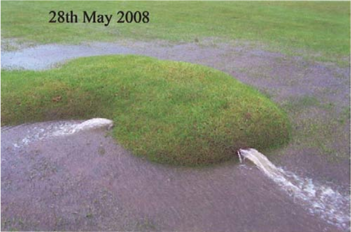
Photograph 7: Heaving of ground on the recreational field due to the water pressure
