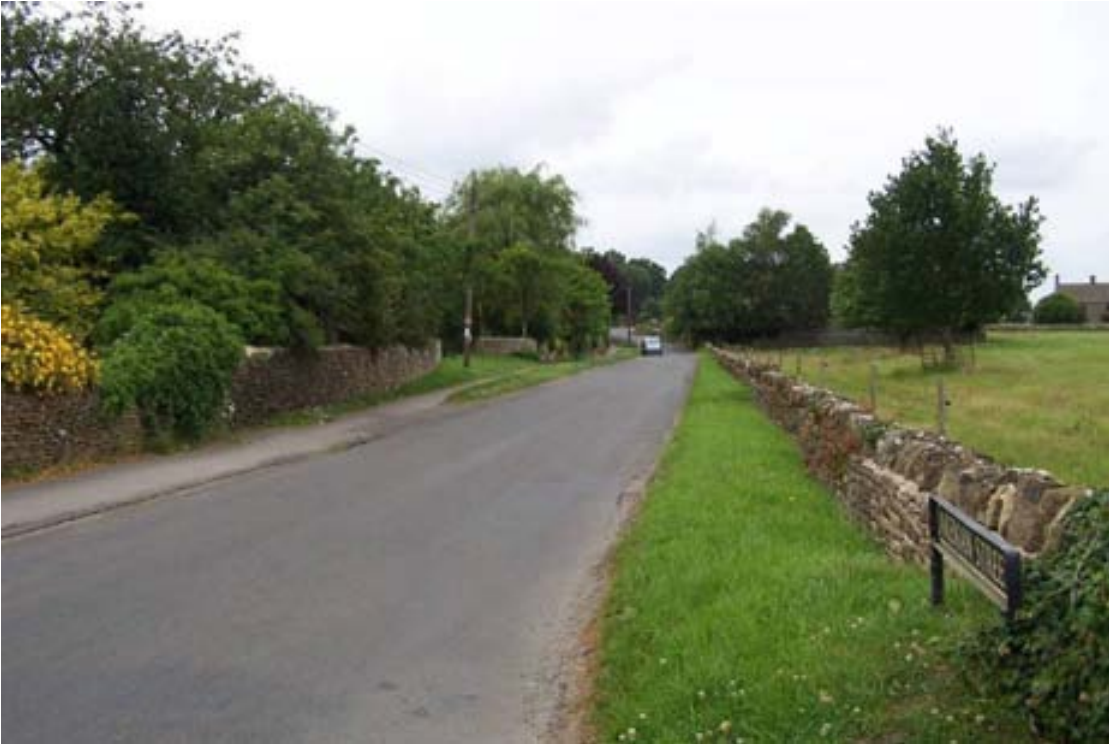
Photograph 17: Akeman Street – looking away from the village towards Square Firs showing a lack of road gullies.
