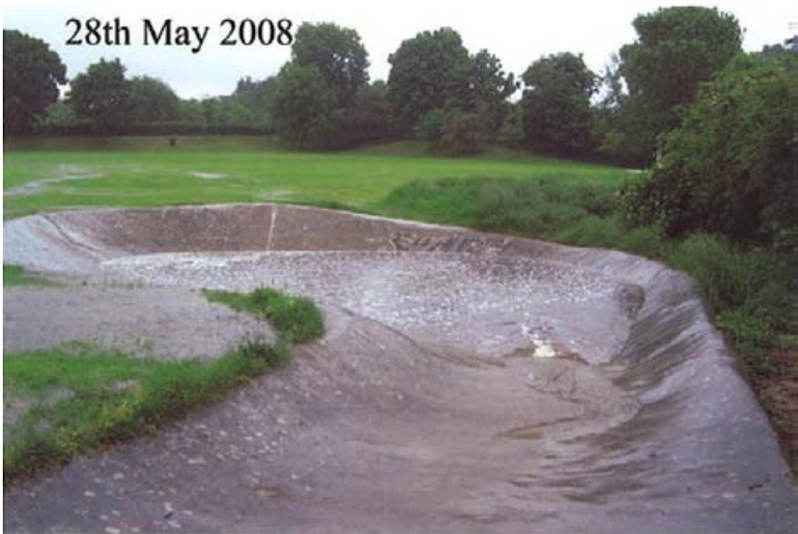
Photograph 6: Flooding at skating bowl at the bottom of the recreational field
