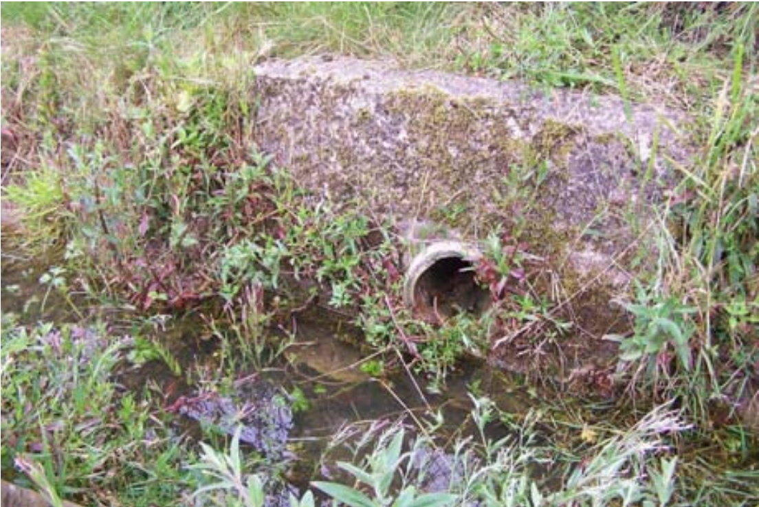
Photograph 13: Outlet from field ditch at rear of property on Park Road at Alma Grove. Drainage connects to highway drainage system on Park Road.
