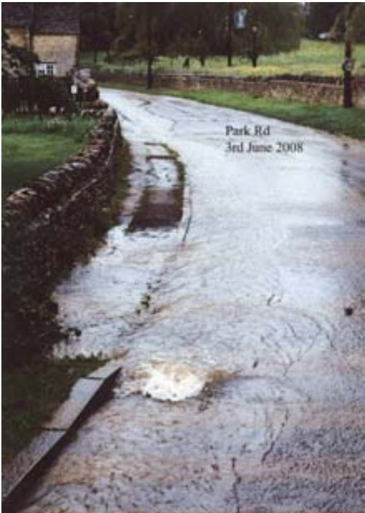
Photograph 16: Water flowing down Park Road at Alma Grove showing the surcharging of road gullies.
