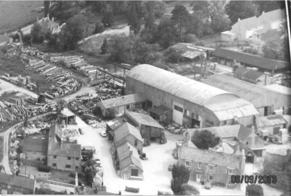
Figure 2: Aerial view of Alfred Groves and Sons Estate circa 1970
