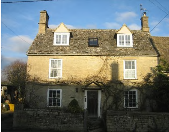
Sunnyside, Shipton Road (note: dormers were added in 2012)
