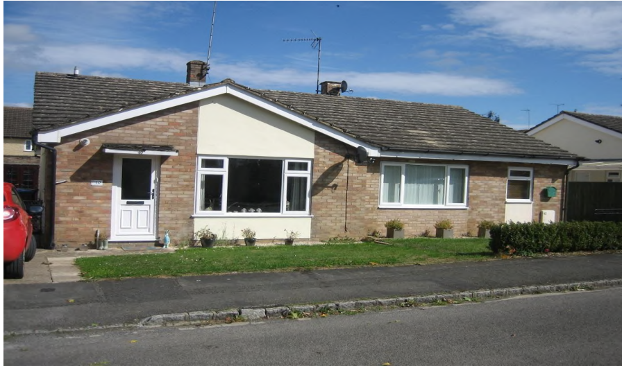
A typical semi-detached bungalow on Wychwood Drive, part brick and part render, with open plan front gardens, designed to look like one property, the house to the right having its entrance to the side gable.
