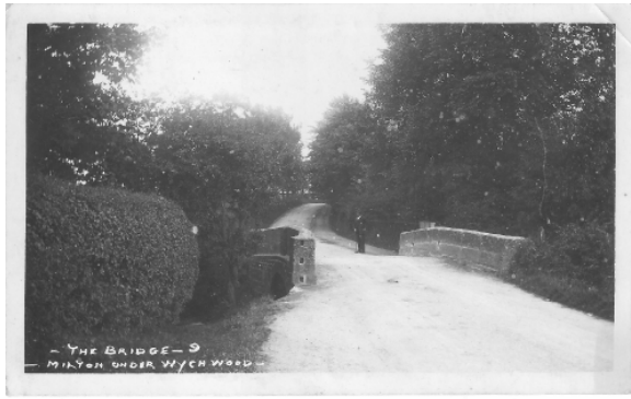
The bridge over Littlestock Brook in a photograph of circa 1920.
