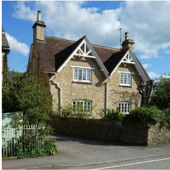
Figure 8: 25 High Street, late 19 th Century House
