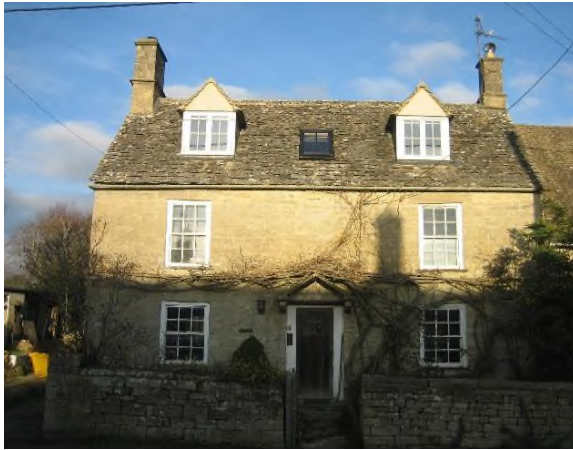
Sunnyside, Sipton Road (note: dormers were added in 2012).
