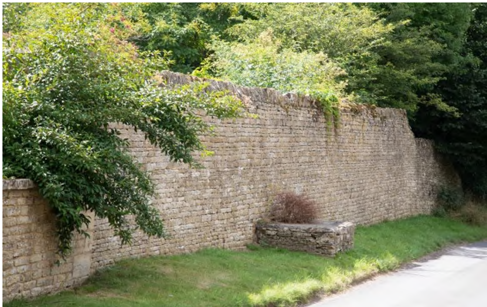
Example of Upper Milton's extensive use of dry-stone walling, and its green verges instead of pavements.
