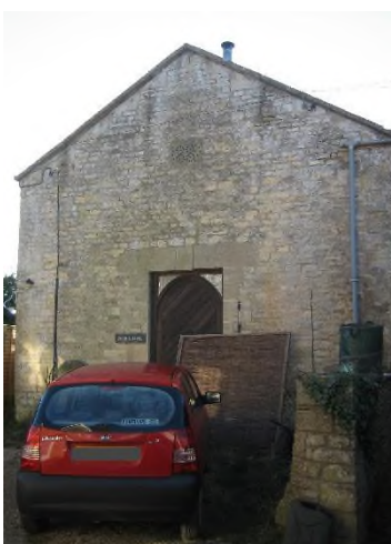
Former Zoar Strict Baptist Chapel, The Terrace 1841/1883.
