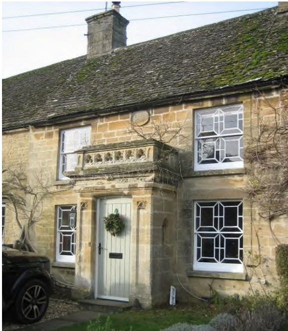
Stone Porch, has date stone of 1725, with unusual Chippendale style sash windows.
