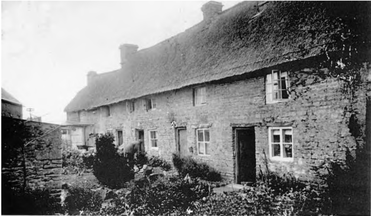
Terrace of cottages on The Square. This row is still in place, though now upgraded and whereas they once consisted of one up one down dwellings, they are now merged into fewer individual dwellings, and once thatched roofs have been replaced with slate or concrete tiles.
