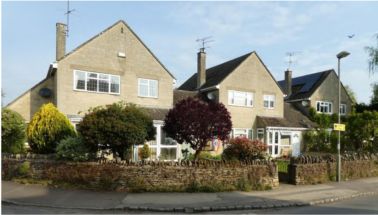
Link-detached houses on Poplar Farm Close present repeating gabled frontages to the High Street.
