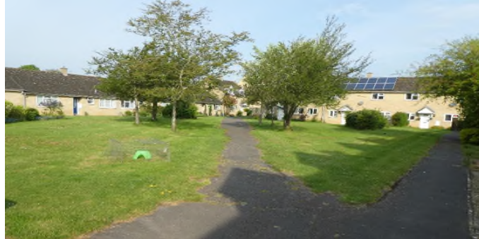
A housing mix of two storey and single storey terraces around an inner garden court between Ansell Way and Fettiplace.
