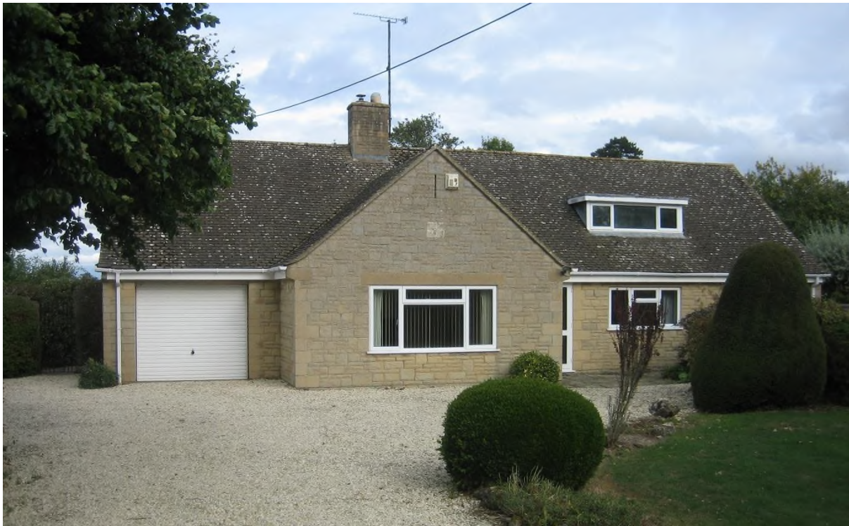
A characteristic bungalow from the 1960s, this one on the Bruern Road from 1966.
