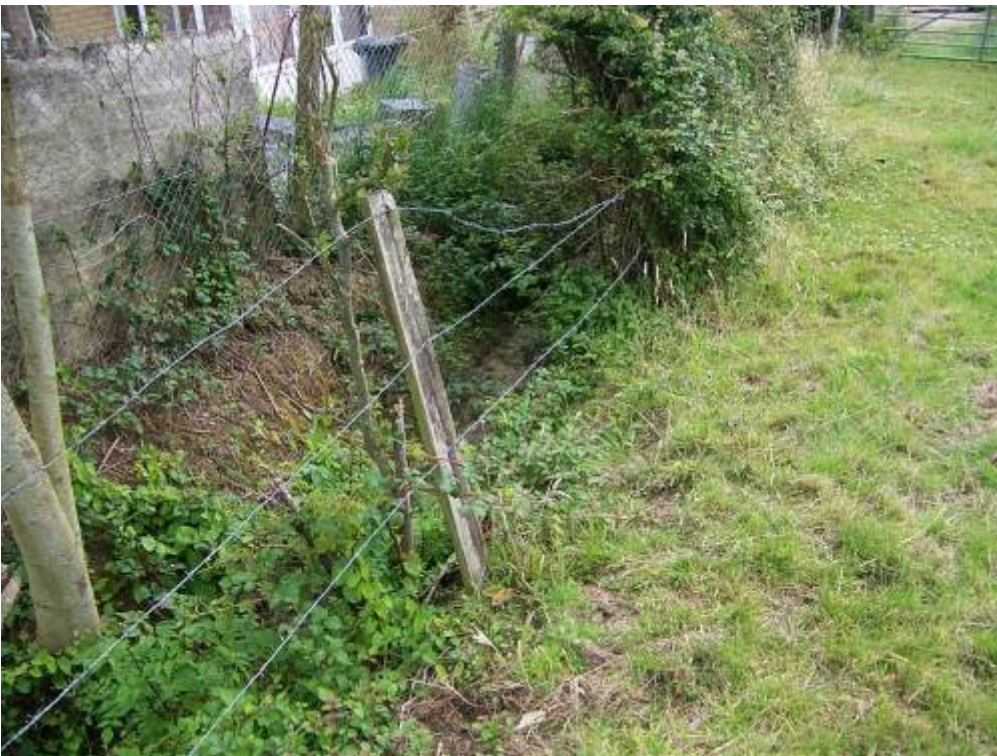
Photograph 21: Poorly maintained drainage ditch
