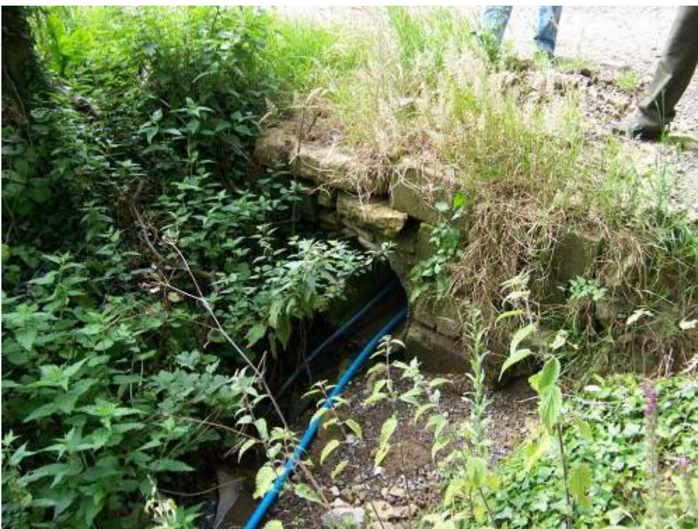
Photograph 15: Larger culvert running along Golden Lane in a north westerly direction
