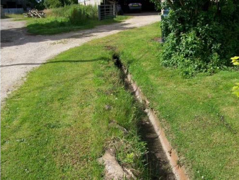
Photograph 4: Blocked drainage ditch along Roses Lane
