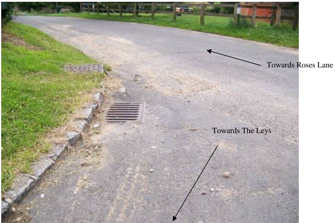
Photograph 17: Gully slightly raised on the corner of road which leads up to The Leys
