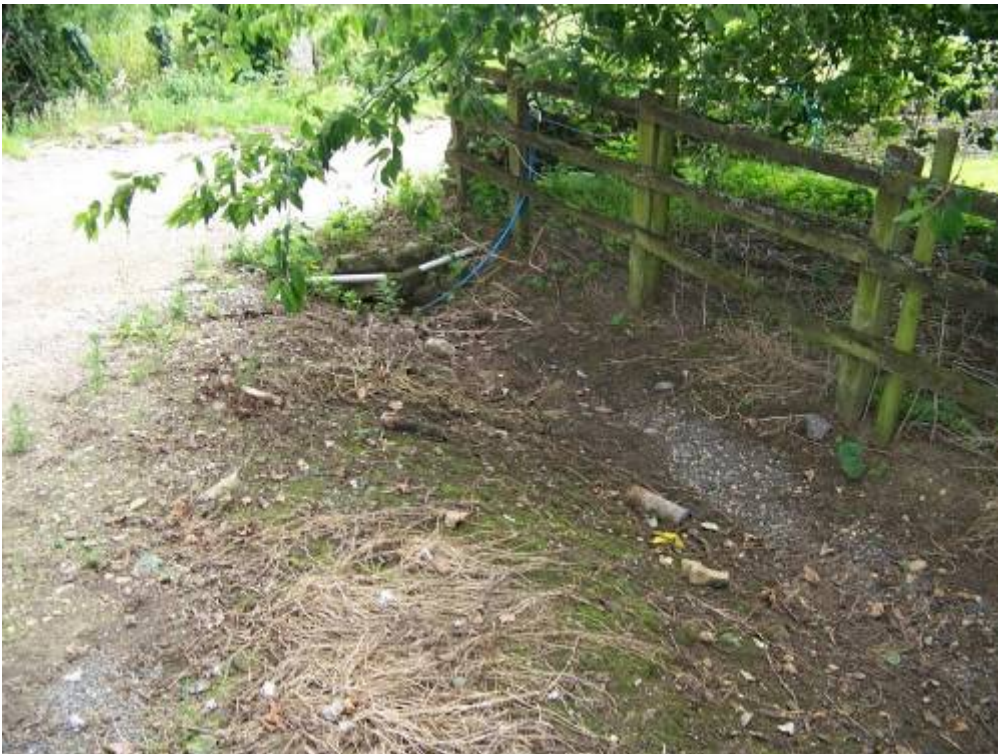
Photograph 14: Culvert at the bottom of fields adjacent to Golden Lane
