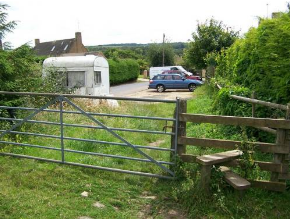
Photograph 23: Water comes off fields and drains through gateway towards The Leys
