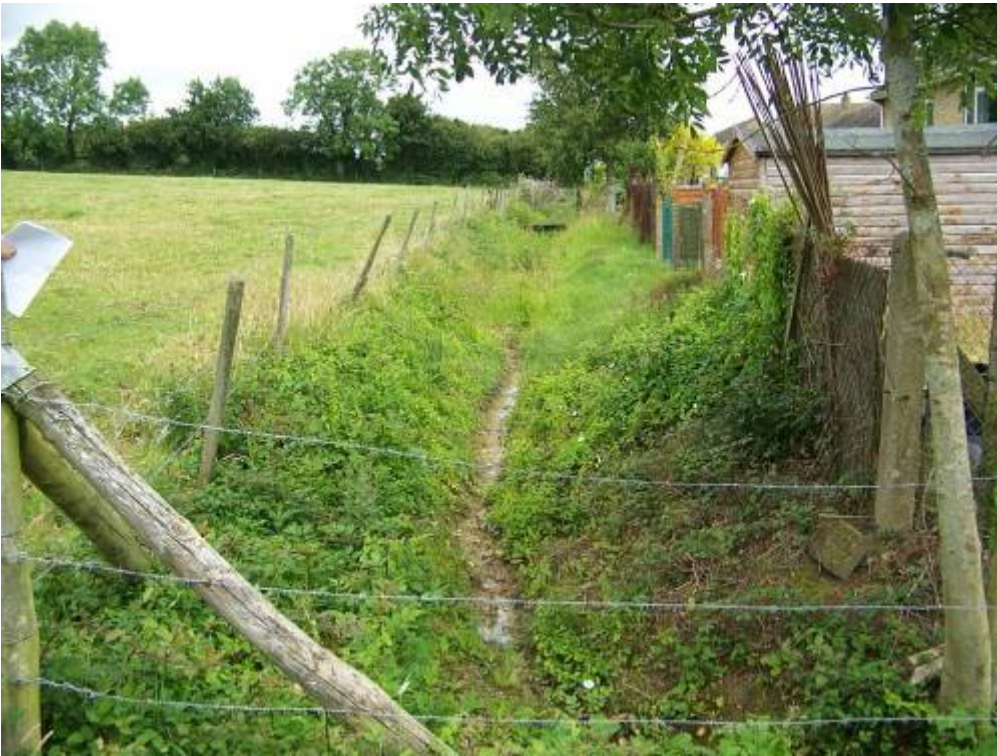
Photograph 21: Poorly maintained drainage ditch
