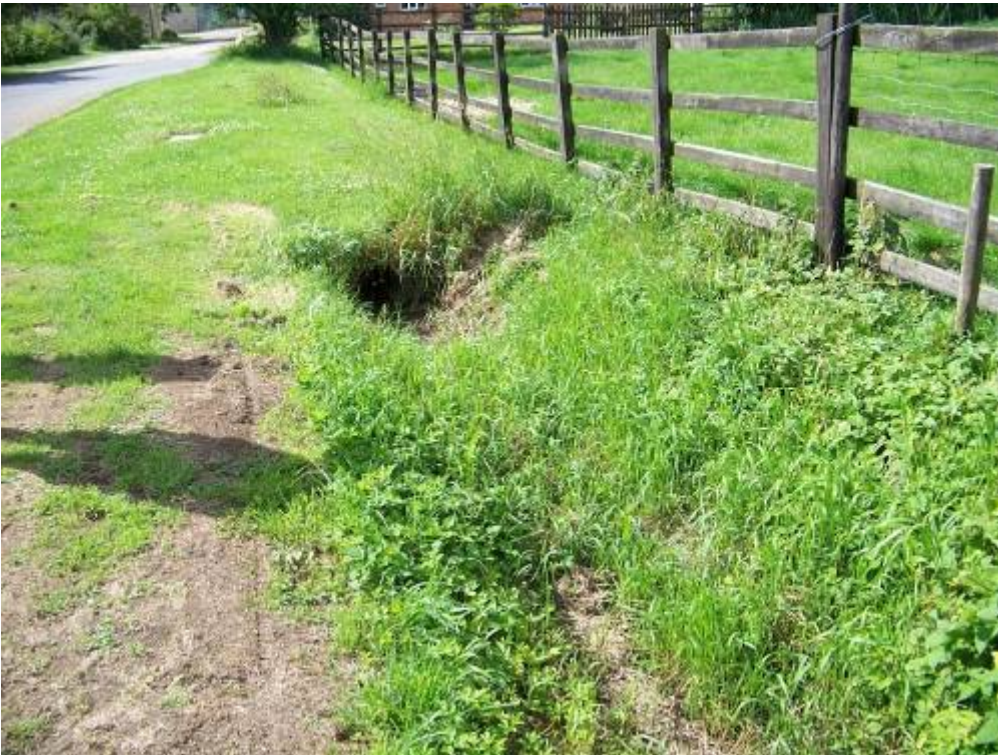
Photograph 6: Overgrown drainage ditch along Roses Lane
