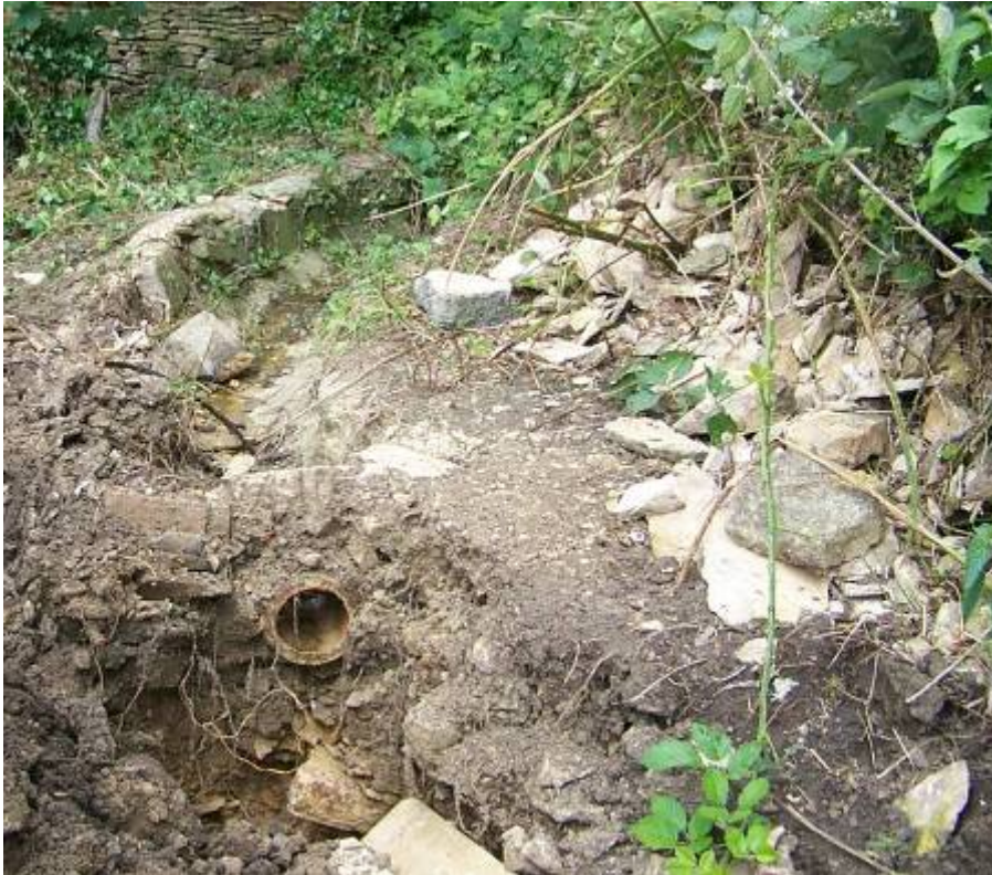
Photograph 25: Culverted watercourse by Chapel Lane
