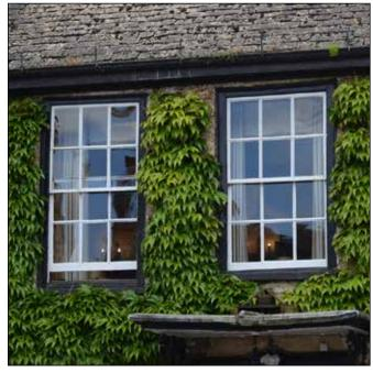
Fig. 2 Traditional vertical sliding sash windows
