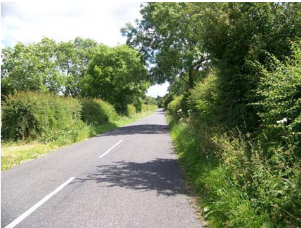
View down High Street to village from B4022 – note steep gradient, lack of road drainage
