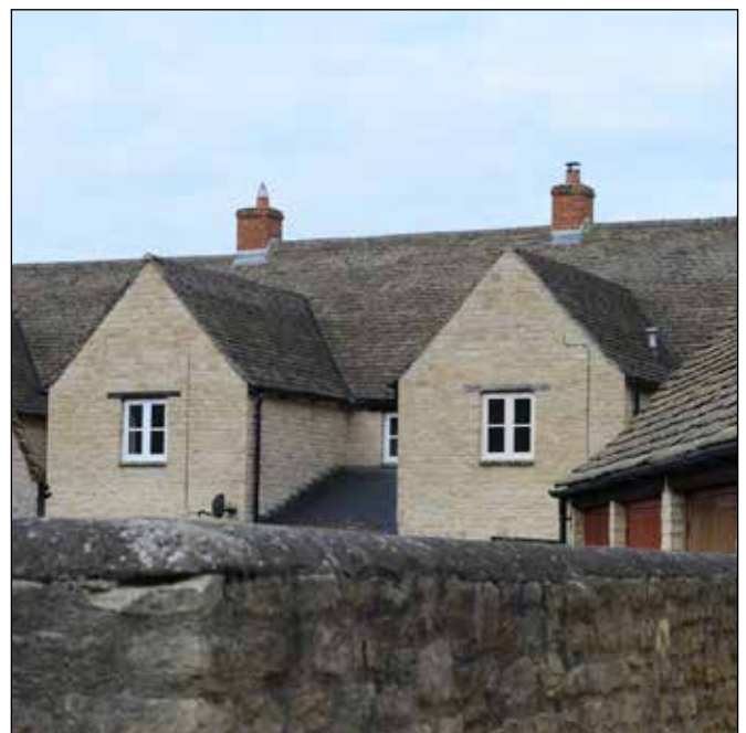
Fig. 3 Two-storey rear projecting gabled extensions
