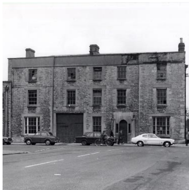
Fig. 7 The former Crown Hotel, demolished to create Langdale Gate
