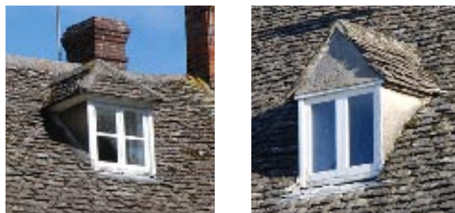
Fig. 13 Traditional, local gabled and hipped dormers
