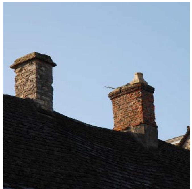
Fig. 10 Stone and brick traditionally used for chimneys
