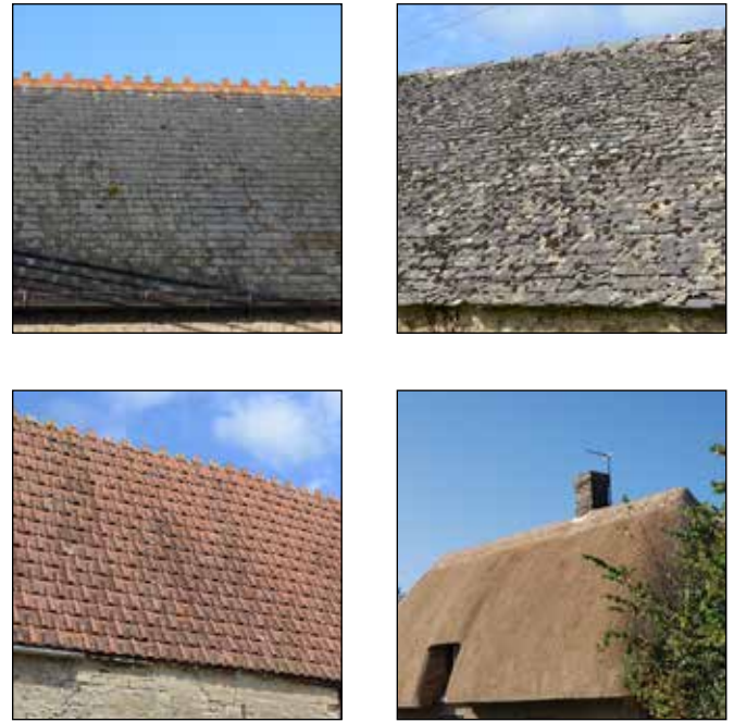
Fig. 3 Welsh slate, stone slate, clay tile and thatch
