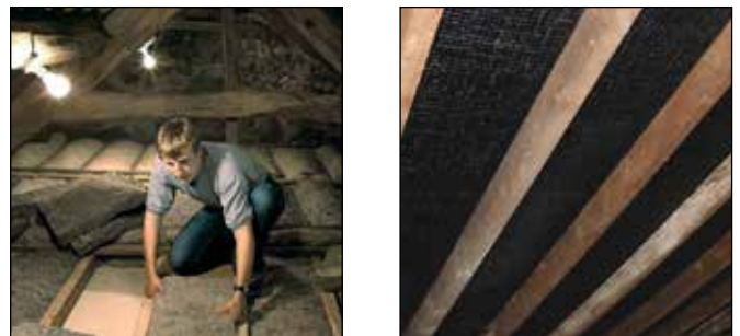
Fig. 6 Insulation can be laid between joists or rafters
