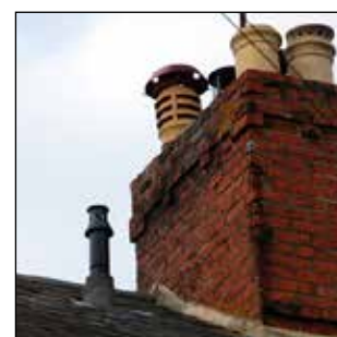
Fig. 11 Combi-condenser boiler, and flue next to chimney
