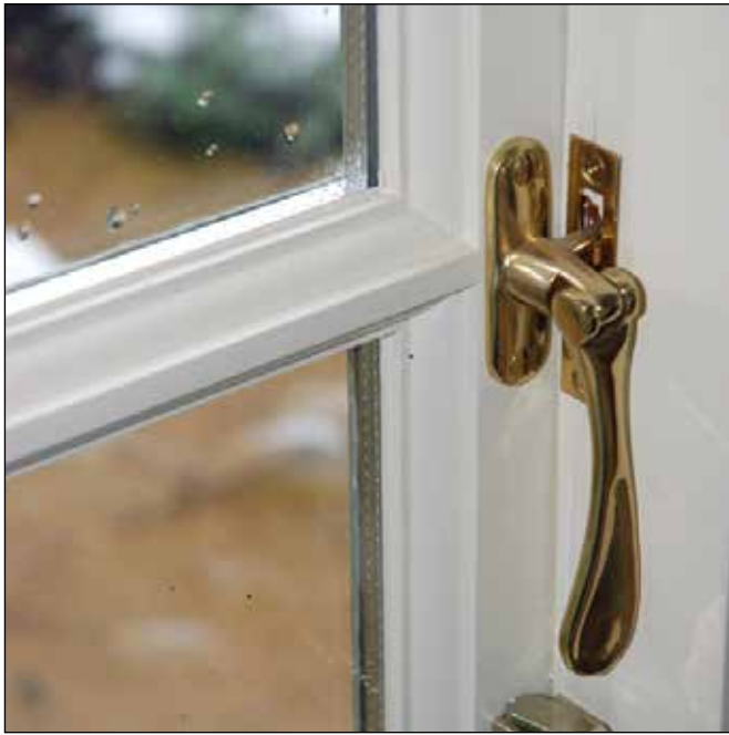
Fig. 9 Slim double-glazing with well detailed glazing bar
