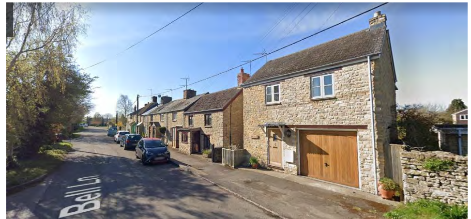
Terrace in Bell Lane including a later addition of Lilly Lodge as an excellent example of the use of traditional detailing © Google 2021
