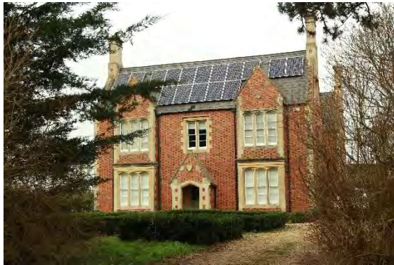
Manor Farmhouse Notable 19th century building (formerly Cassington House). Red brick building with stone quins (often used to reflect higher status buildings) of two storeys with attics and a slate roof.
