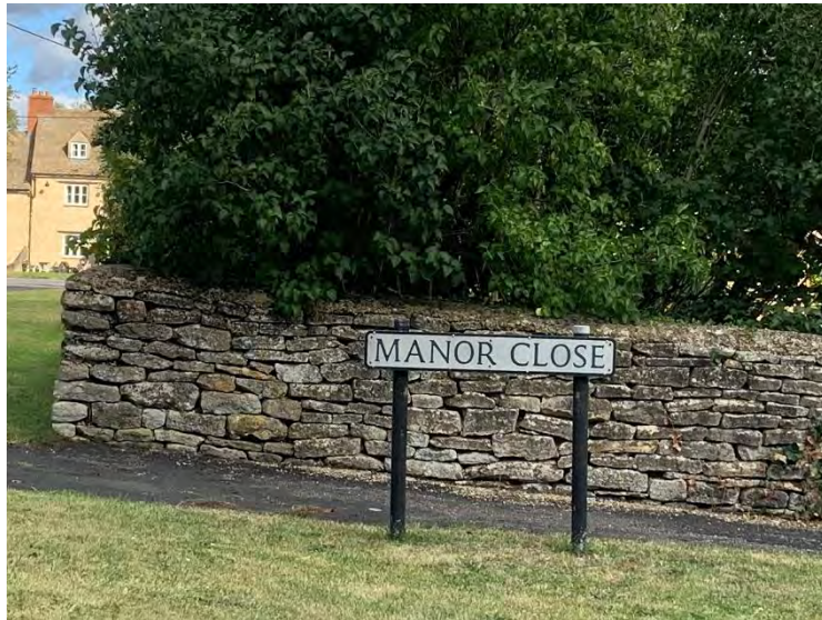
Drystone wall at Manor Close with the Chequers Inn terminating views into the Conservation Area party seen in the background
