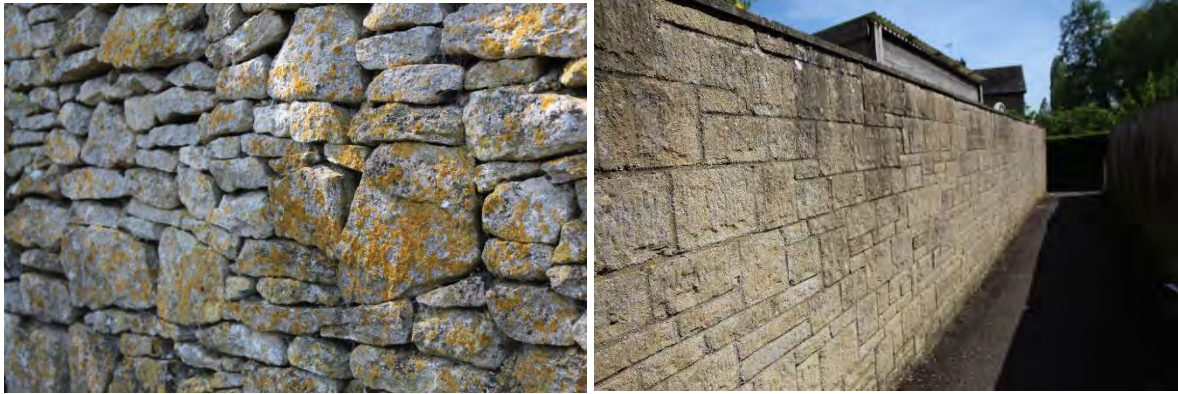
Figure 27. The strong contrast in construction and wildlife friendliness of old dry stone walls compared to modern built stone walls in Cassington. Both photos from the vicinity of the foot path from the Upper Green to the Lower Green. The old walls have many living spaces for insects, slow worms and other organisms and a strong growth of lichens.
