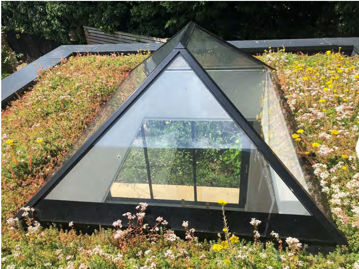
Figure 41. Green roof on building in Cassington village. Not only does this provide advantages in terms of cooling of the building but it also provides flowering plants for pollinators such as bees.
