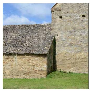
Fig. 6 Existing traditional materials should be retained
